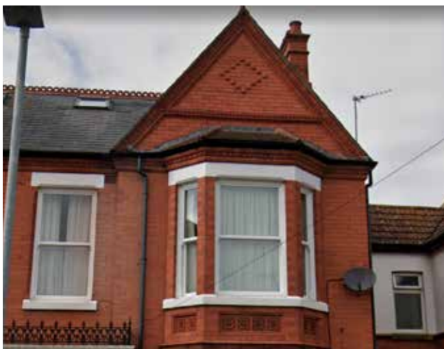
Brickwork details on Highfield Park
